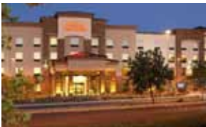
A.R. Mays Construction
